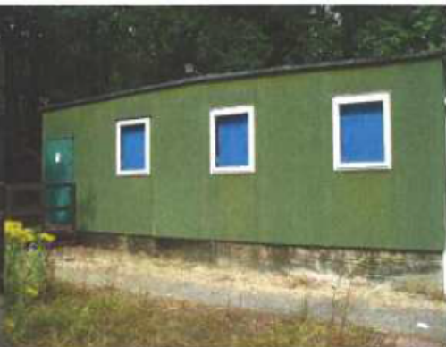
Port Cabins South-East Elevation
