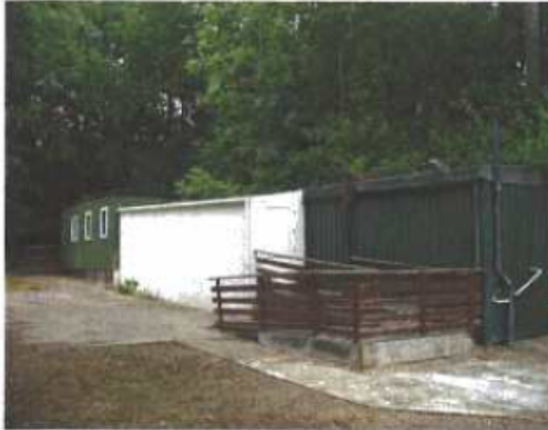
Port Cabins South-East Elevation
