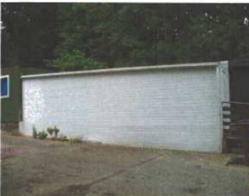
Port Cabins South-East Elevation
