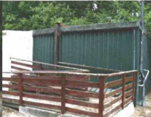
Port Cabins South-East Elevation
